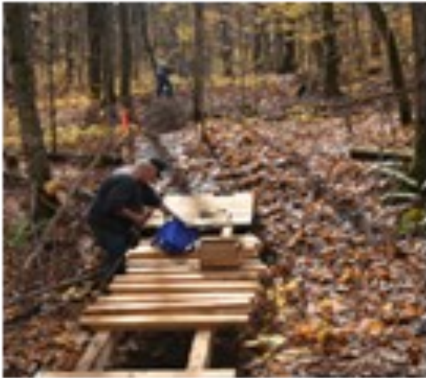
Brian Barbour working on one of the many new bridged walkways
